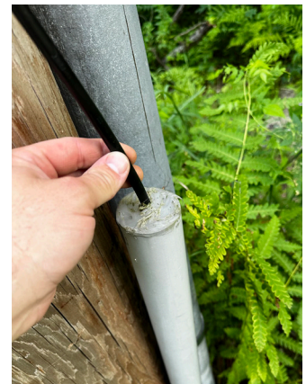
Closeup of 1.25" conduit with communications wire. Wire moves freely when pulled.
